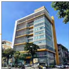
PHNOM PENH MAIN BRANCH 18 December 1993
